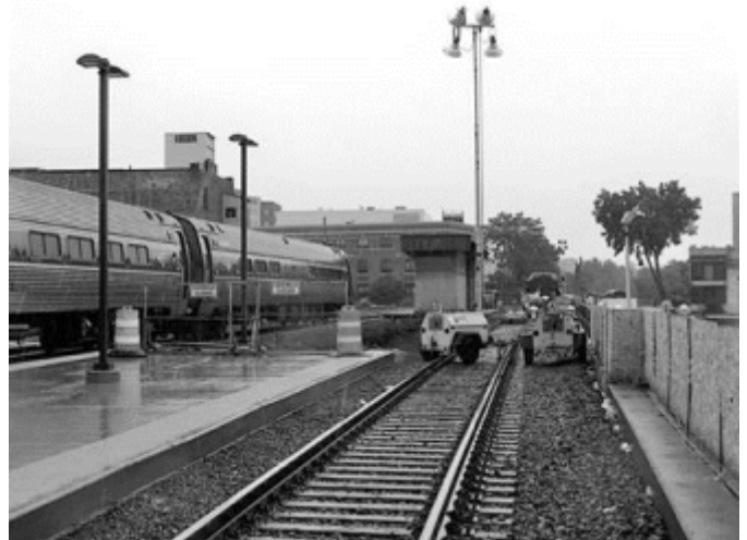
View of station construction from temporary station
